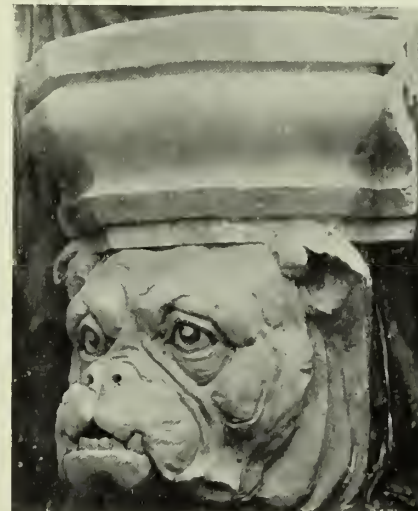
DETAIL FOR YALE BOAT HOUSE, NEW HAVEN, CONN. South Amboy Terra Cotta Company, Makers. Peabody & Stearns, Architects.
